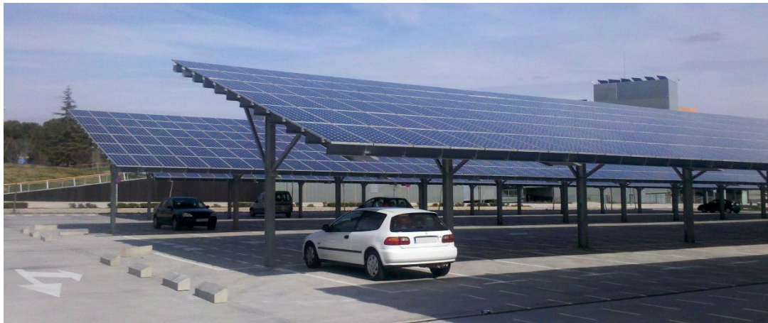
Figure 25 PV panels used as roofing over a parking space represents another form of multi-use of land [21]
