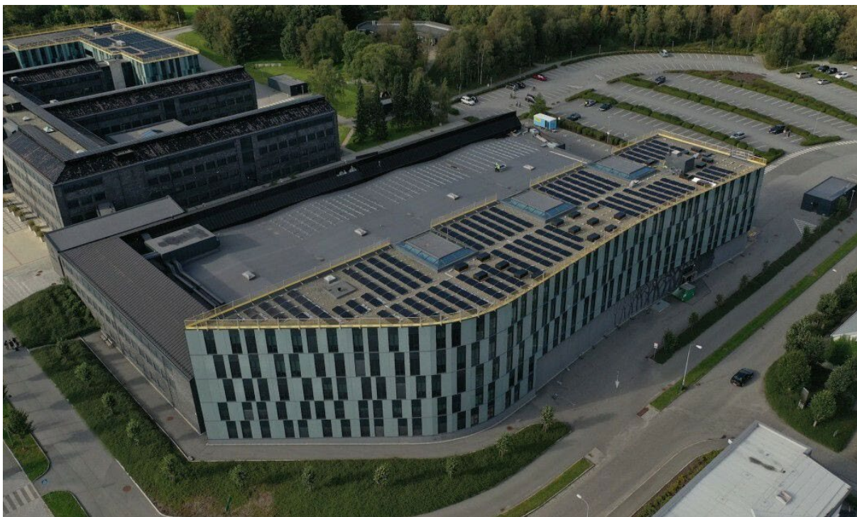
Figure 19 Oljedirektoratet in Stavanger is an example of a building with roof and wall integrated PV panels. Both the grey and black panels on the wall are PV panels [11].
