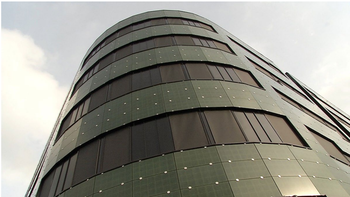
Figure 27 Using PV panels as the facade and roof material is a perfect example of highly efficient multi-use of land. Incorporating solar into the building materials could make them pay for themselves during the building's lifetime. Also, the panels take up no additional space. The picture is of the building "Solsmaragden" in Drammen [22].
