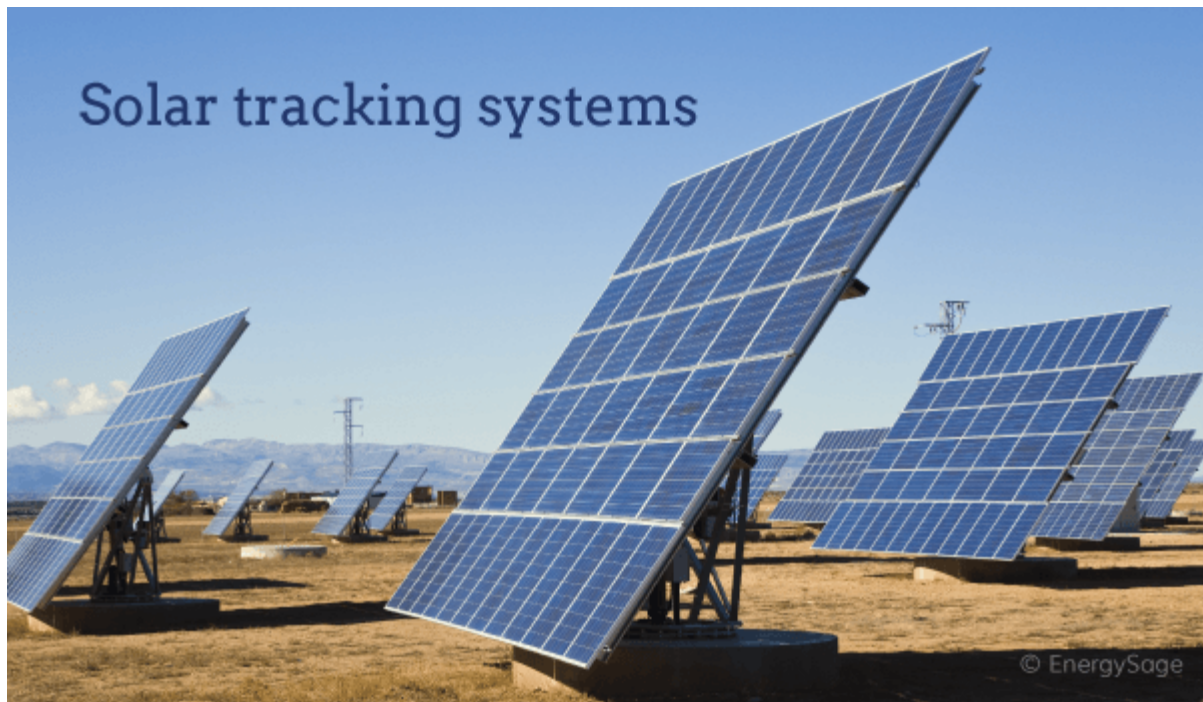
Figure 21 Solar tracking provides the maximum possible power produced, but it comes at a higher investment and maintenance cost [15]
